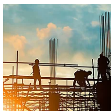
Building the Advanced Manufacturing
